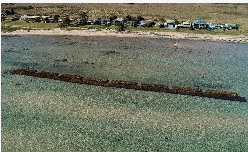
Shellfish reef breakwater with two adjacent modules after construction
