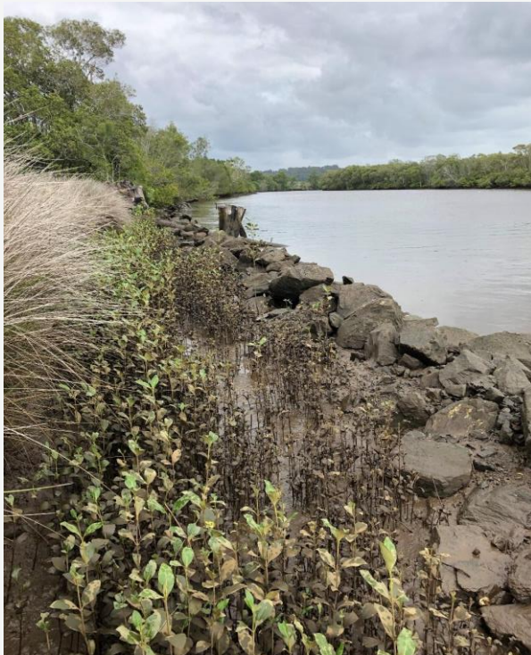
Rock fillet, with first year mangrove recruits, Ballina NSW
